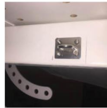
8. Tighten screws. Repeat steps 3-8 on the other side.
