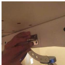
4. Hold up loop for placement, keeping it in a horizontal alignment, close to the bottom edge of the metal frame.
